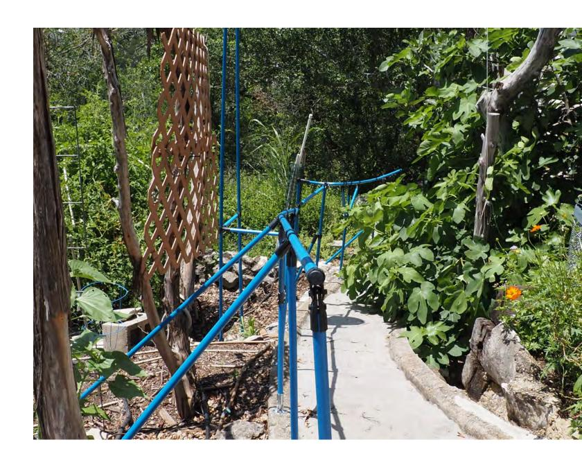
Close up from the bottom of the ramp. All of the top bars of the handrail, where we grab the handrail for support, are wrapped in heat shrink. All vertical posts and bracing pieces are painted to match.
