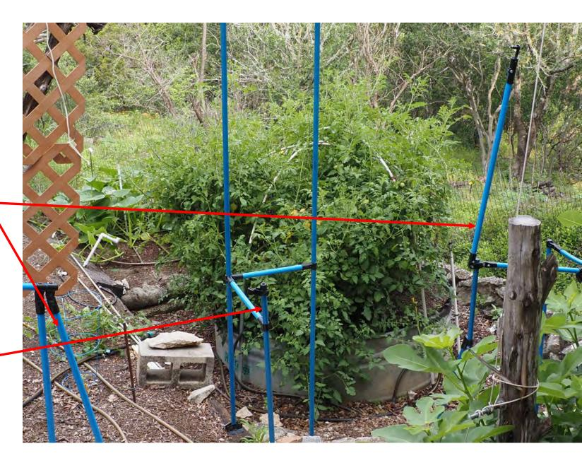
To create the hinge for the section that swings up I used an adjustable 180-degree connector. Selftapping screws through the connector permits leaving the 5 mm hexhead bolt slightly loose to allow for motion.
