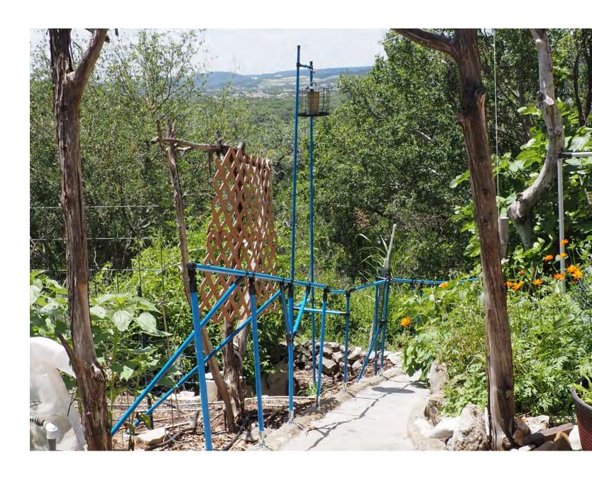
This access was provided by creating a vertical hinge for two adjacent sections of the top rail seen here in the open position.
