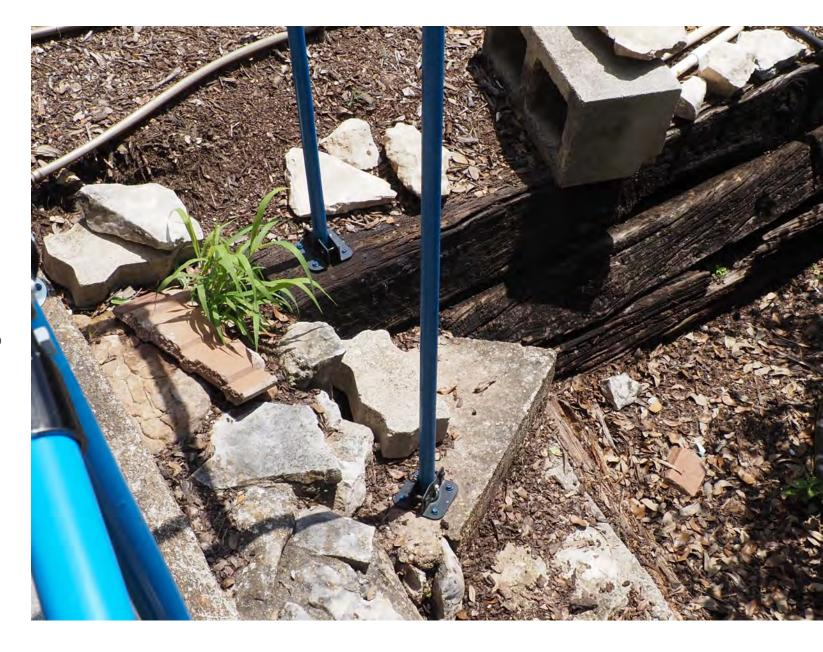
Adjustable angle flanges and 45-degree connectors were used to support the vertical posts for the angled braces.
