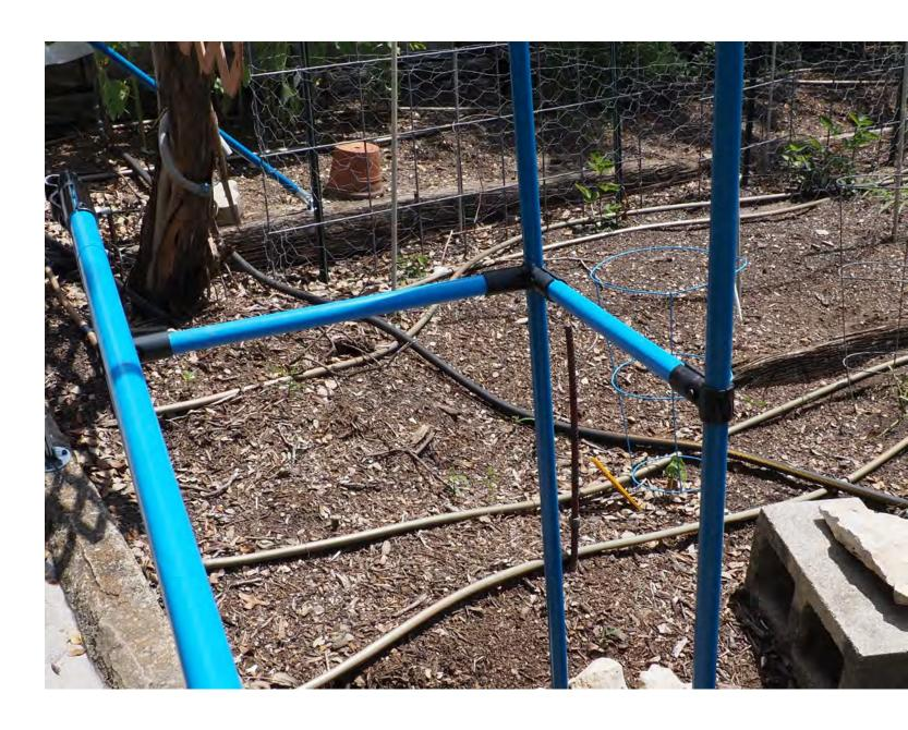
Flange connectors into concrete or a railroad tie supports the vertical sections. I drilled a 1-inch diameter hole into the railroad tie to slip the conduit down 8 inches for extra support.
