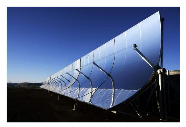
The parabolic trough operates by focusing the sun's rays on the central tube. The assembly is oriented north and south, and tracks the sun as it moves east-to-west by varying its tilt-angle.
