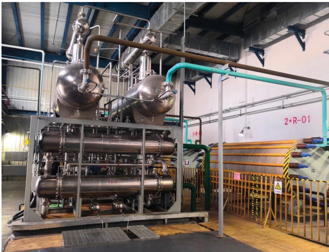
Figure 9: John Cockerill's 5 MW-Alkaline Stack (right) Connected to its Balance of Plant
