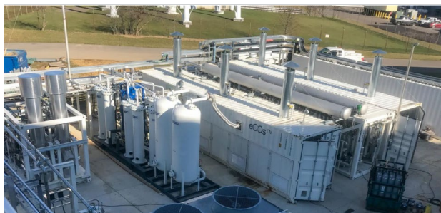
Figure 21: Topsoe eCOs™ Electrolyzers at a DeLille Oxygen Co. Site 42,43
