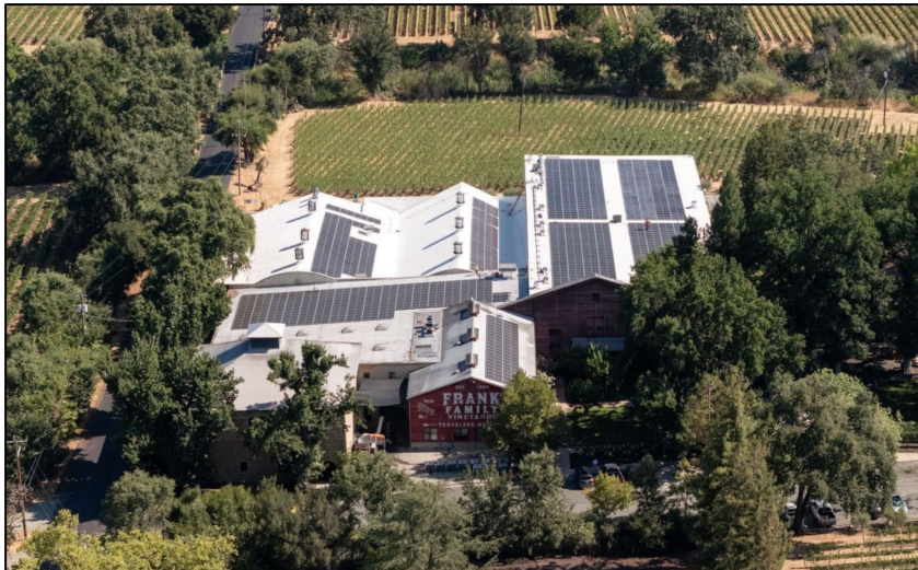
Frank Family Vineyards Solar Array - Photo Courtesy of Frank Family Vineyards
