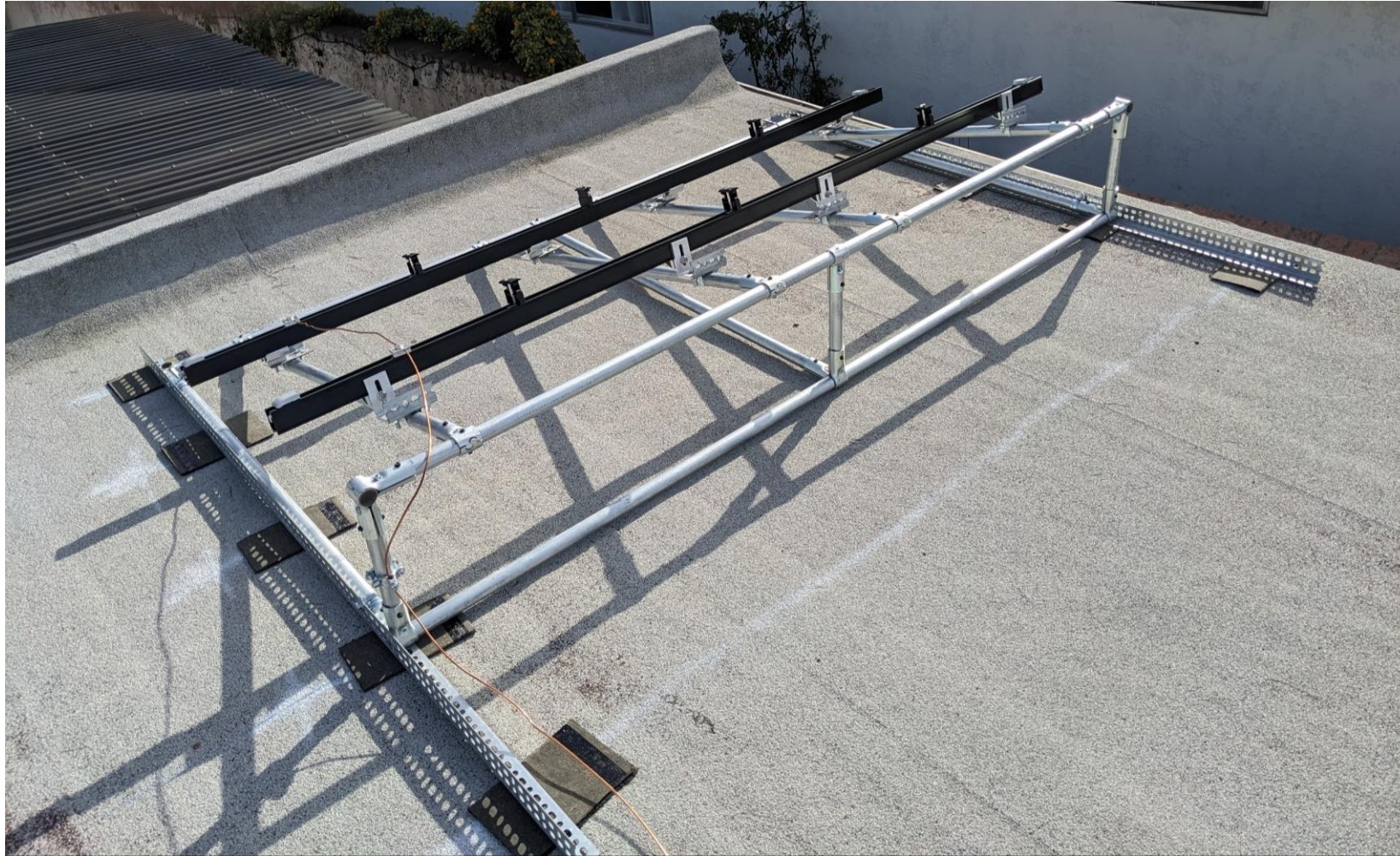
Final solar panel array frame set in place
