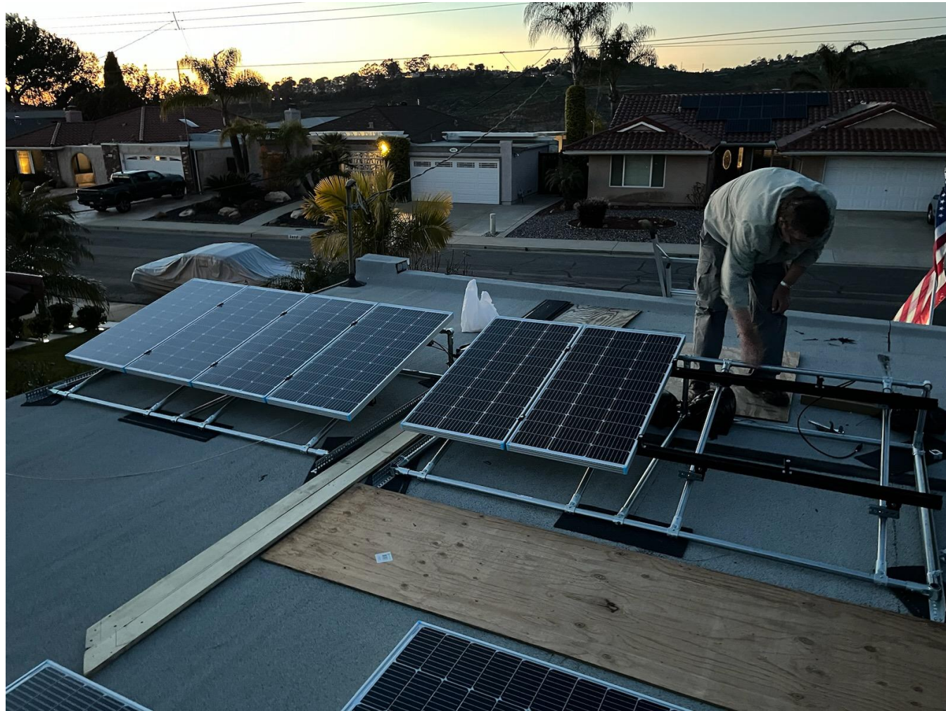
First two solar panel arrays being completed
