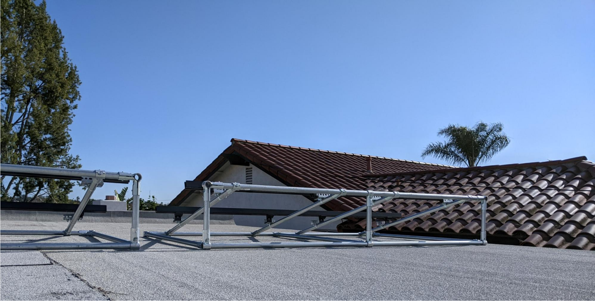
First two solar panel array frames set in place
