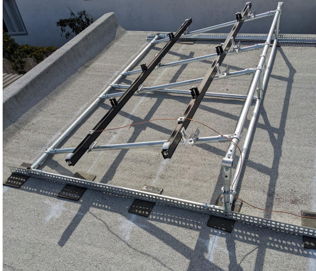
Final solar panel array frame set in place
