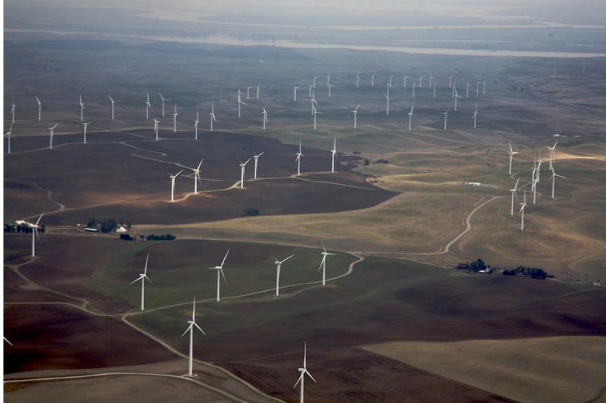
An early 2017 image of part of the Altamont Pass Wind Resource Area showing the many small turbines that populated it then. Image by Marli Miller, Geologic Time Pics.
