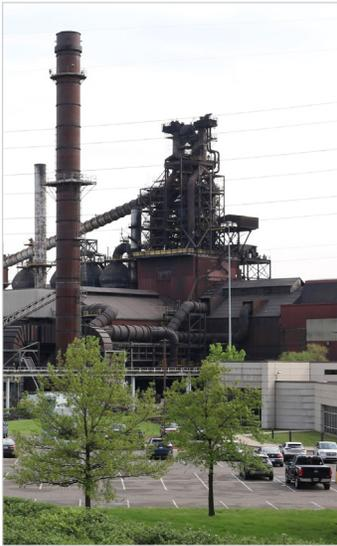
Dearborn Works relies on a centuries-old technology for crude iron production from mined iron ore: the blast furnace (Figure 2). The crude iron output of Dearborn's sole blast furnace is then refined into crude steel in either of two basic oxygen furnaces. Next, the hot, liquid crude steel is tailored into specialty steel compositions in two ladle metallurgy furnaces, before passing to a set of slab casters. See [GET THE FACTS: How is steel made?](#)
