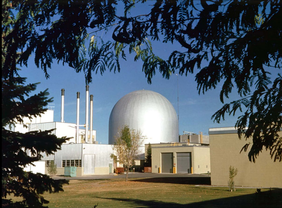
Starting in 1964, the Experimental Breeder Reactor-II proved the concept of fuel recycling and passive plant safety characteristics.
