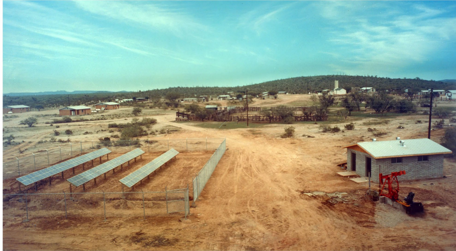
Schuchuli village in southern Arizona with solar panels on the left in November 1978.
