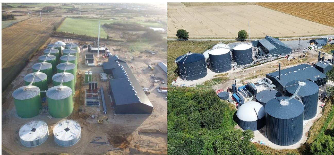
Figure 8 SBS Kliplev (to the left) is approx. 8.5 ha and has an annual production of 48 million Nm 3 of biomethane, whereas Solrød biogas (to the right) is approx. 2 ha and has an annual production of 11 million Nm 3 biomethane [23, 21]
