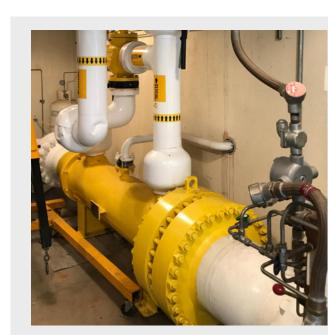
The U-Tube configuration of the type BEU allows it to handle differential thermal expansion since the bent tubing is inherently free to expand.
