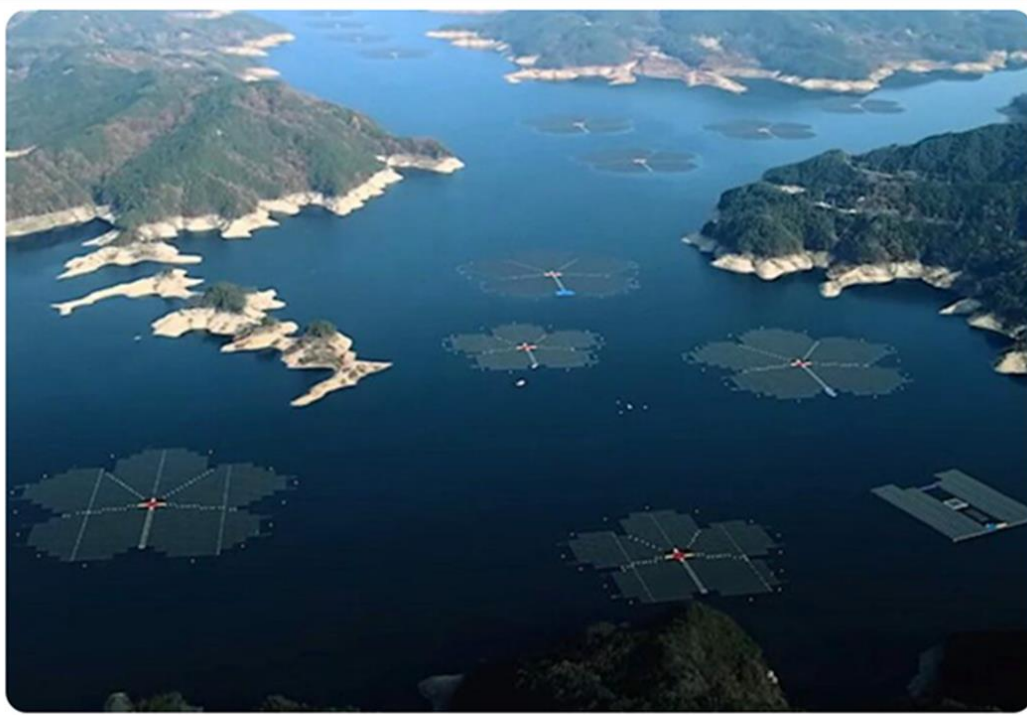
The 17 giant photovoltaic flowers on the 12-mile-long Hapcheon Reservoir in South Korea generate 41 megawatts
