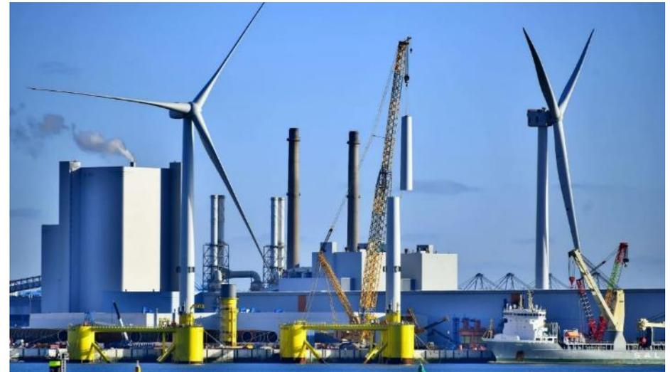
**Figure 39 Floating offshore wind turbine final assembly taking place at port. Photo of the Kincardine Offshore Wind Farm project courtesy of Principle Power.**
