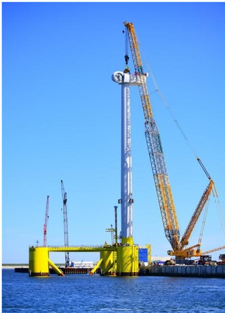
**Figure 40 A landside crawler crane lifting a nacelle onto a floating substructure. Image courtesy of Port Pictures / Danny Cornelissen. All rights reserved.**
