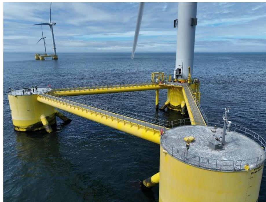
**Figure 22** Semi-submersible floating substructures used at the WindFloat Atlantic project. *Photo of the WindFloat Atlantic project courtesy of Principle Power/Ocean Winds.*
