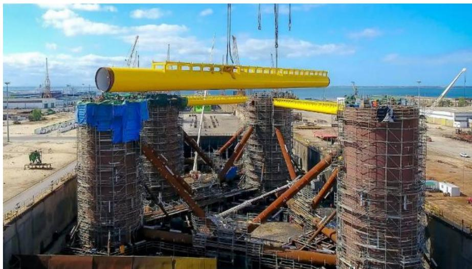
**Figure 23** The final assembly of the primary structure of a steel semi-submersible floating substructure. *Photo of the WindFloat Atlantic project courtesy of Principle Power/Ocean Winds.*
