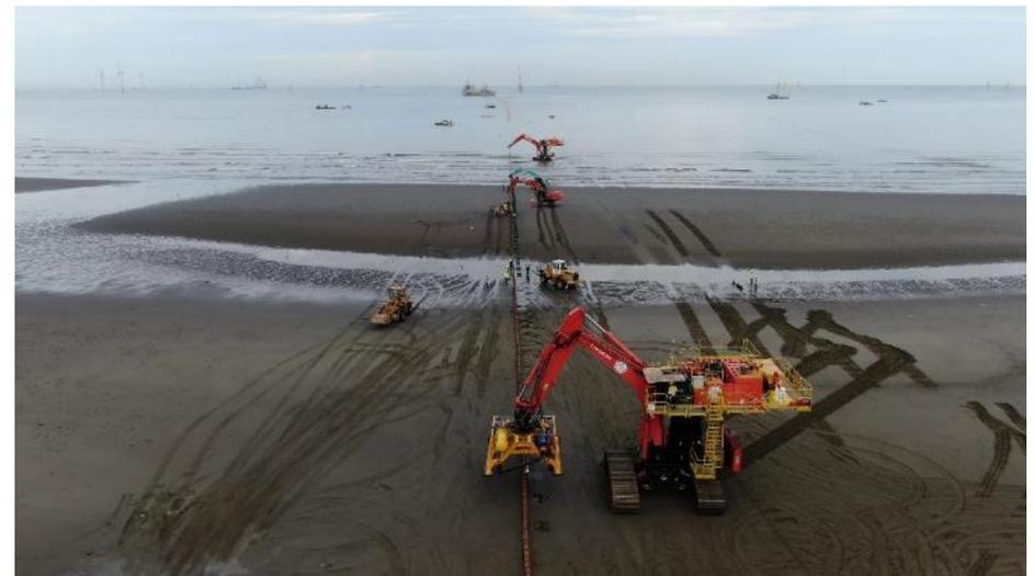
**Figure 34 Offshore export cable transitioned to shore. Image courtesy of Jan de Nul. All rights reserved.**
