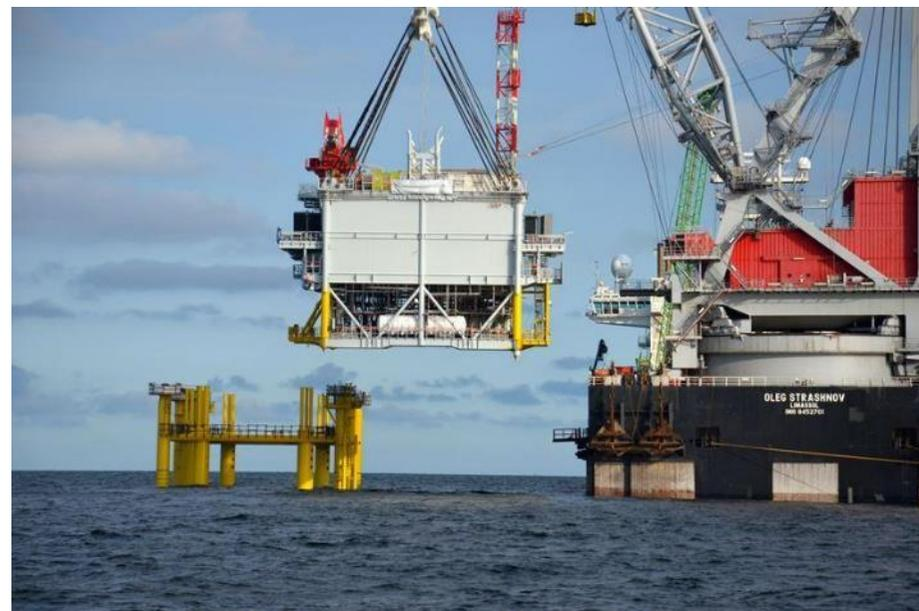
**Figure 33** Topside structure of an offshore substation being lifted onto a jacket foundation. *Image courtesy of ScottishPower Renewables. All rights reserved.*
