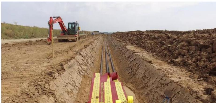
**Figure 36 Onshore export cable trenching process.** *Image courtesy of Ørsted. All rights reserved.*
