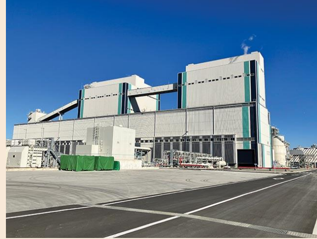
The 650-MW Yokosuka Thermal Power Station Unit 2 came online in December 2023 uses USC technology
