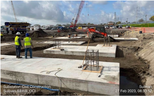
In-process foundations on top of piles for bus supports (left) and transformer foundations (right)
