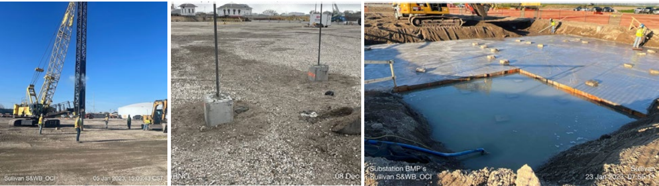
Left: concrete pile driving. Center: installed concrete piles, prior to foundation caps and foundation installation. Right: preparation for installing grouped foundation on top of piles with mud mat and pumps to dewater.
