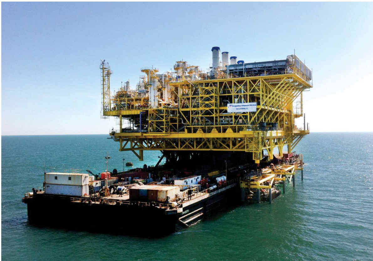
FIGURE 21.8 EXAMPLE OF A FLOAT OVER TOPSIDE INSTALLATION
