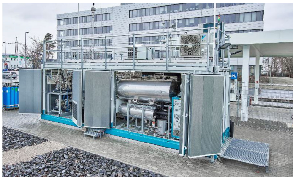
Figure 3. Dehydrogenation unit of Hydrogenious at the hydrogen refueling station of H2 MOBILITY Germany in Erlangen. [63]
