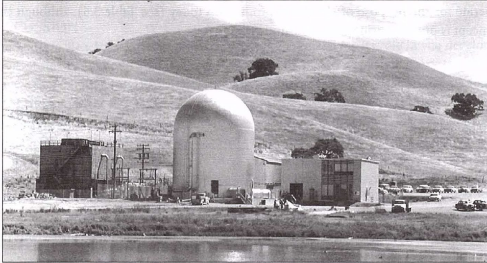
Vallecitos Boiling Water Reactor (VBWR), Pleasanton, California. (Used with permission of GE Hitachi Nuclear Energy.)
