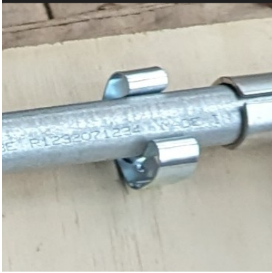
Closeup of the grip clip that holds down the deck to the frame.
